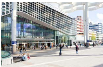
Parking Garage Hoog Catharijne - Utrecht the Netherlands
