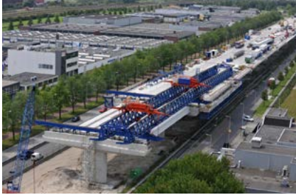
Westrandweg - Amsterdam the Netherlands
