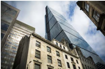
Leadenhall building - London United Kingdom
