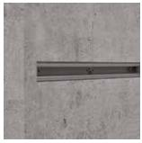
4.) No filler or concrete left overs should be left within the channel slot. Any residue should be scrapped out
