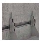
8.) When the connection has been made recommended torque must be used in order to fasten the T bolts
