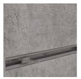
5.) Suitable T head bolts should be inserted into place by placing the narrow side of the head in the slot
