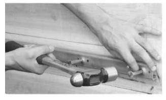
1.) Anchor channels are fixed to form work after careful planning and positioning. Concrete is then cast in to the form work.
