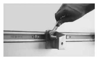
4.) Fixtures are fastened with the T bolts and nuts as shown above. Correct loading and torque values need to be applied in accordance with the allowable loads of the channels and bolts.
