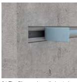
3.) The filler can be pulled out along the length of the channel simply by hand
