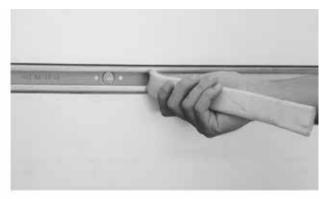
2.) After the concrete is cured, the filler inside the channel, set for the purpose of preventing concrete filling the channel's slot, is removed as shown.
