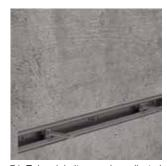
7.) T head bolts can be adjusted along the length of the channel to be in the desired position
